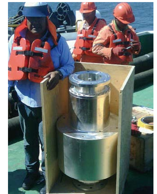
Example of application: Installation of a 8" NTS®-PU
